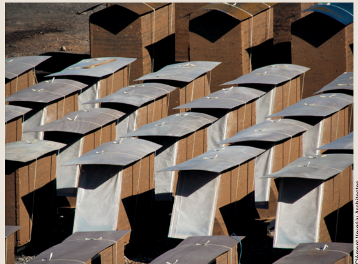
The earth blocks of l’Orangerie in Lyon by Clément Vergély Architectes and Diener & Diener Architekten are air dried and stored near the construction site.
